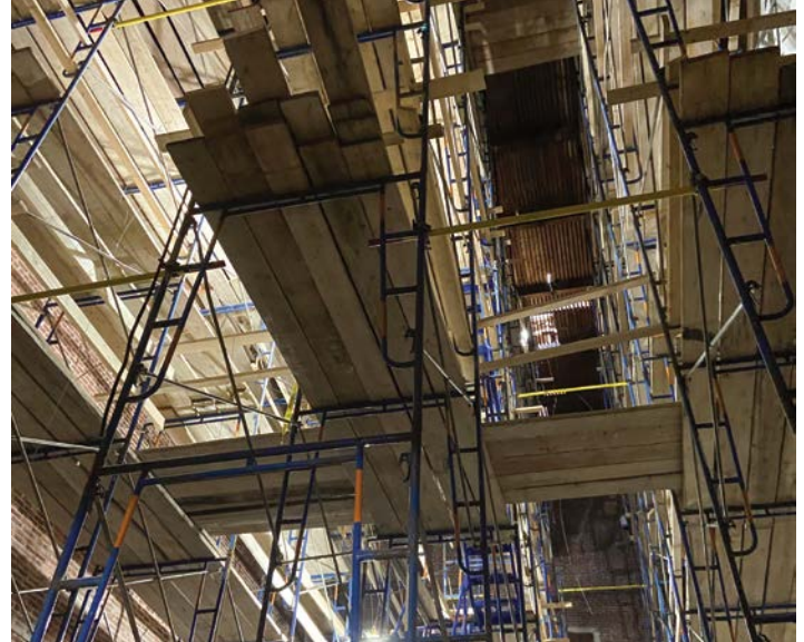
Left: BPS crews are entering the final stages in a massive project to renovate Laconia's famed Colonial Theater. Right: Skyscraper-like towers of scaffolding are required to access the upper reaches of the theater.
