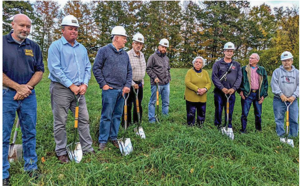
Sanbornton residents, town officials and project team members gathered this past October to celebrate the groundbreaking for the new Town Offices Building.
